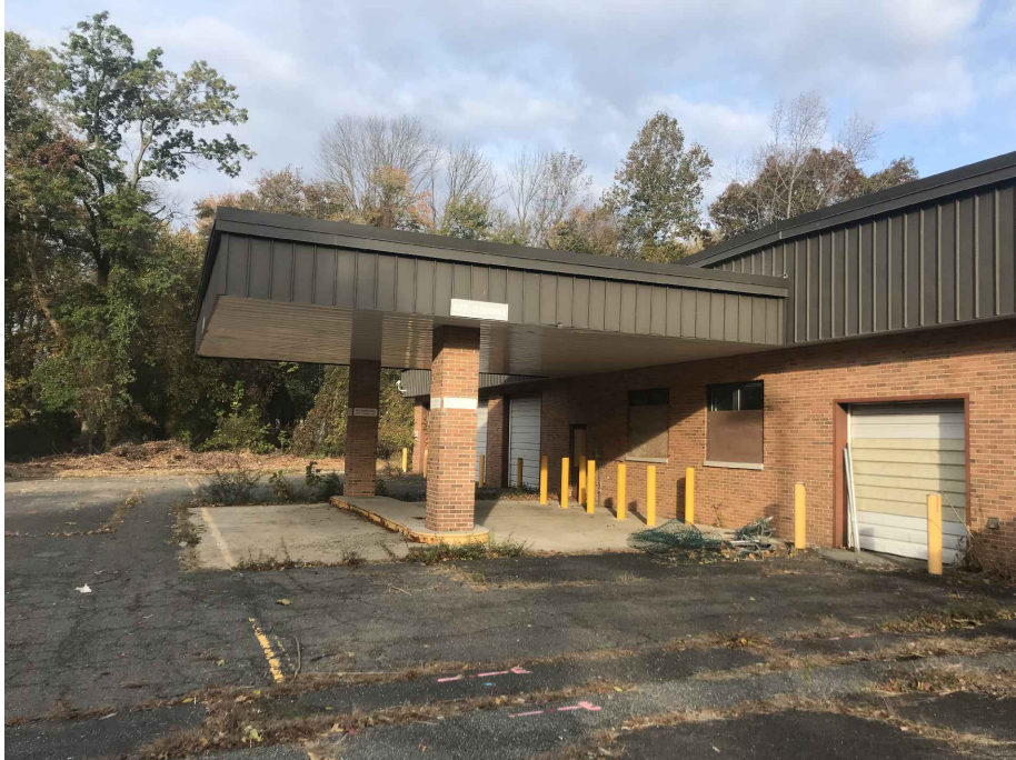
VIEW 5 - STRUCTURE TO BE MAINTAINED
