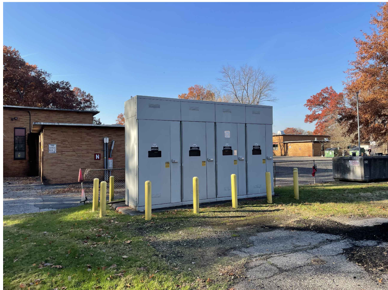
VIEW 37 - TO BE REMOVED
