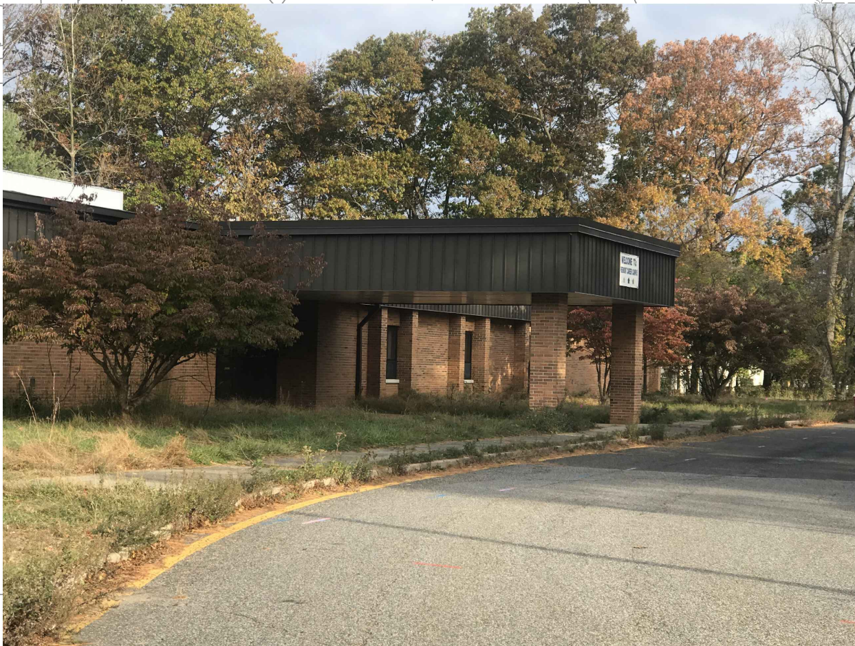
VIEW 12 - STRUCTURE TO BE MAINTAINED
